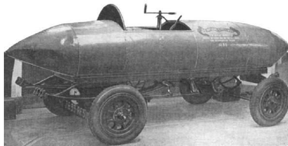
Figure 2. EV called James Contente, which in 1899 achieved an unprecedented speed of 100 km / h[4]
