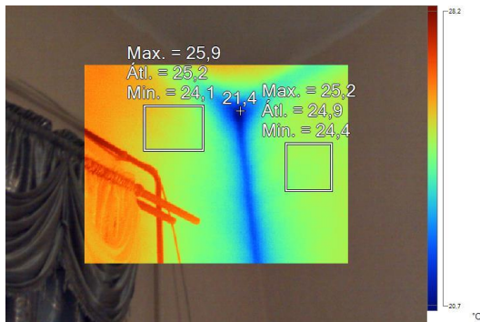
Figure 14. Upper corner, below unoccupied flat, facing to the courtyard
