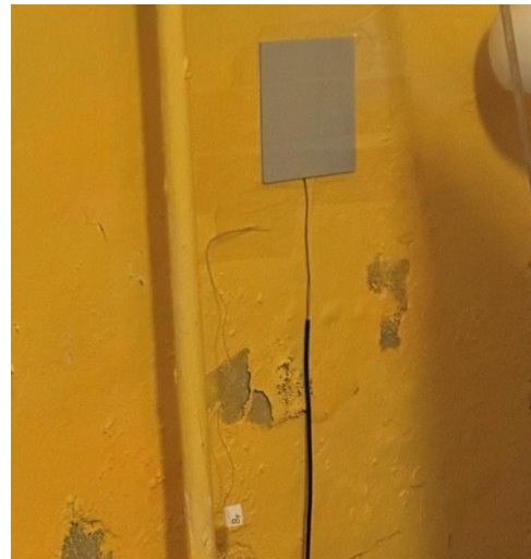
Figure 7. Heat flux meter and temperature sensors installed on the inside
