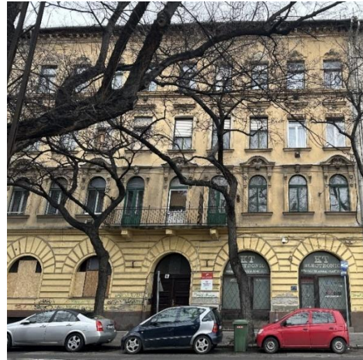
Figure 4. Diószegi Sámuel street 18., facade
