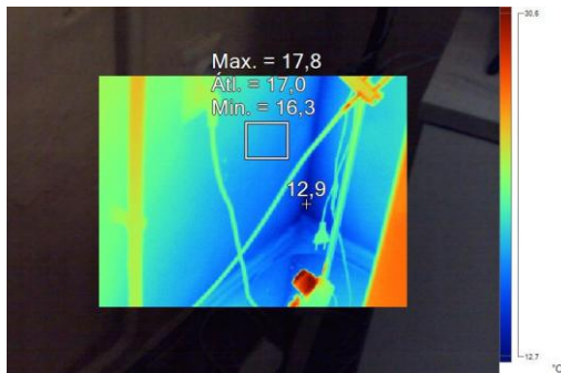
Figure 16. Lower corner, above unheated basement, facing to the courtyard
