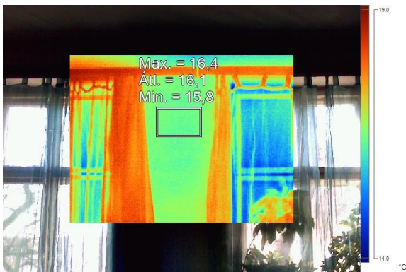
Figure 26. Façade wall, facing the street
