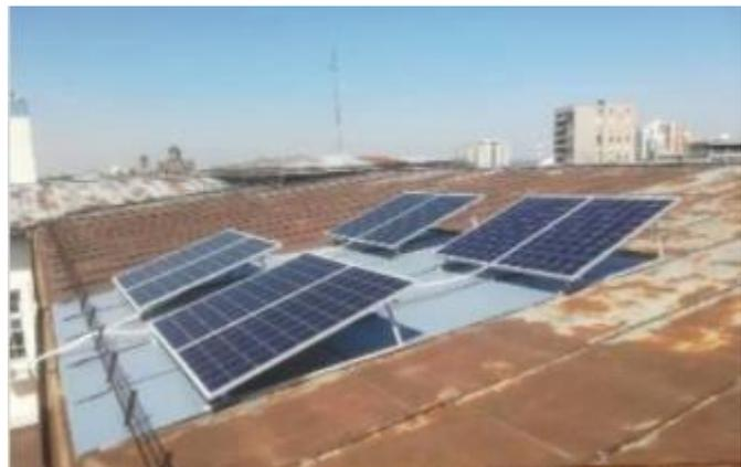
Figure 6: PV panels on the rooftop
