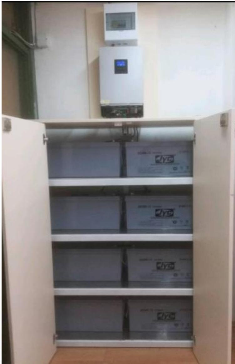
*Figure 7: Safety fuses with converter, batteries and charge controller*
