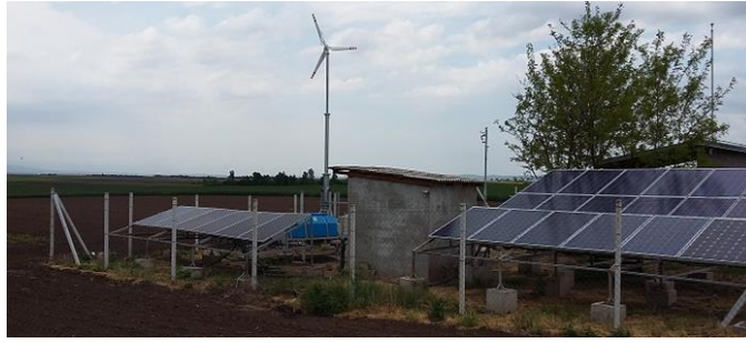
Fig.13. Disposition of the PV power plant (total power 2 \times 12 \times 250W = 6kW ) and wind turbine 0.5kW with mounting pole.
