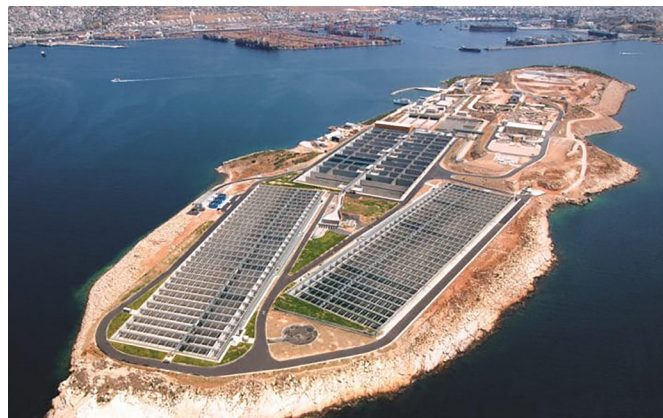
Slika 3.1: Areal view of the Psytalia WWTP [5]
